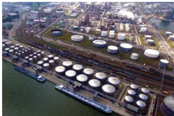
Ergon International's storage terminal located in Antwerp, Belgium
